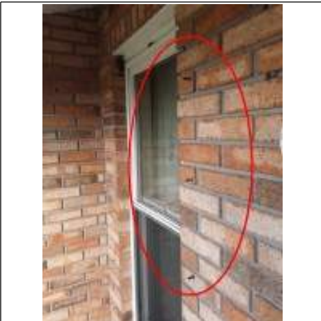
Shutter Wall Studs
